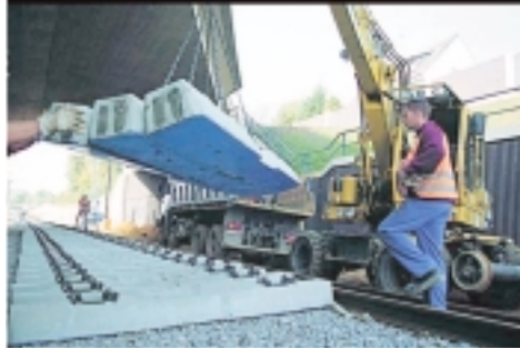
Laying sleepers with Sylomer elastic sleeper pads
