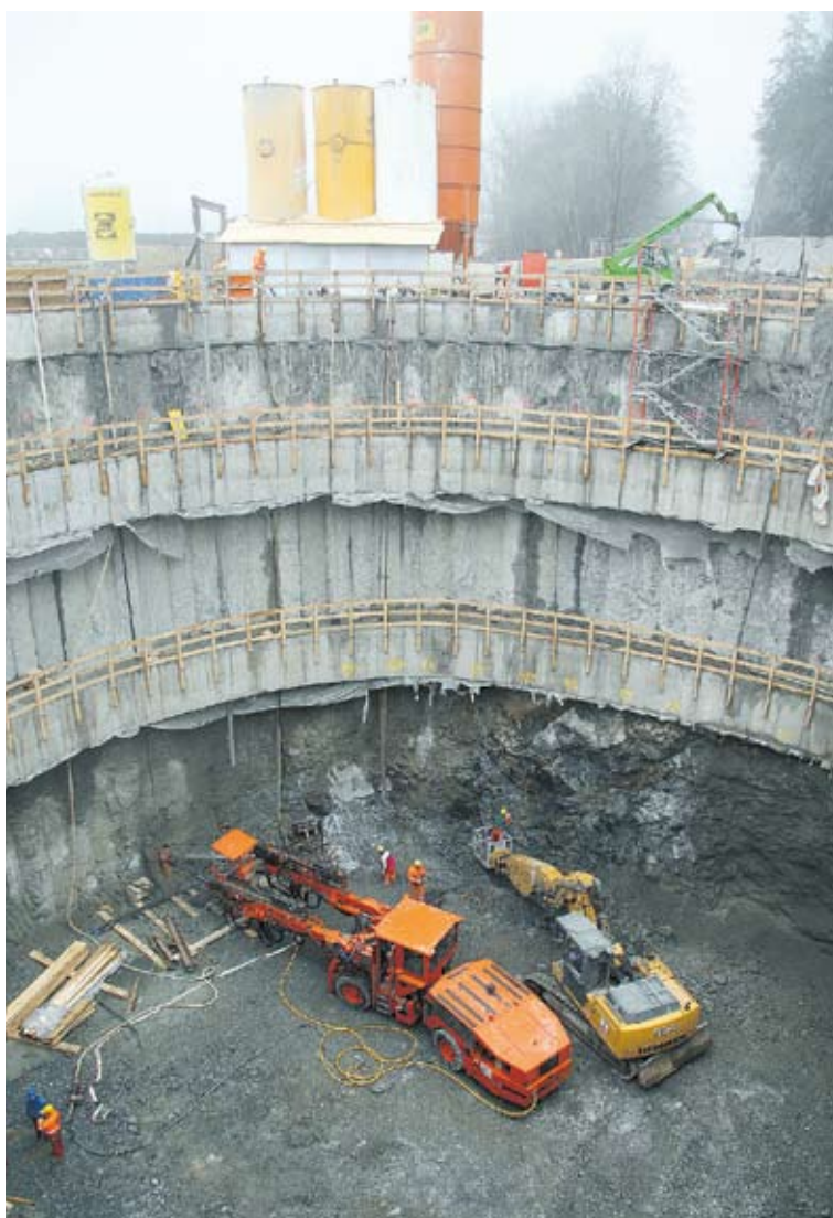
The shaft at Matzen before arrival of the tunnel boring machines.
