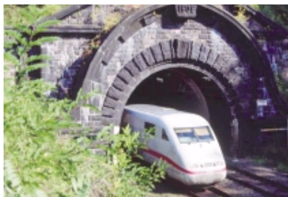
A second tunnel is to be built to relieve the old Schlüchtern Tunnel
